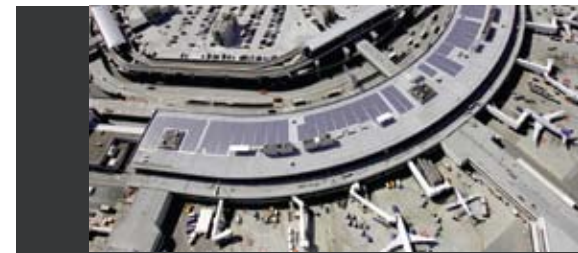
Thanks to its Suntech solar power system, San Francisco International Airport is one of the "greenest" airports in the U.S.
